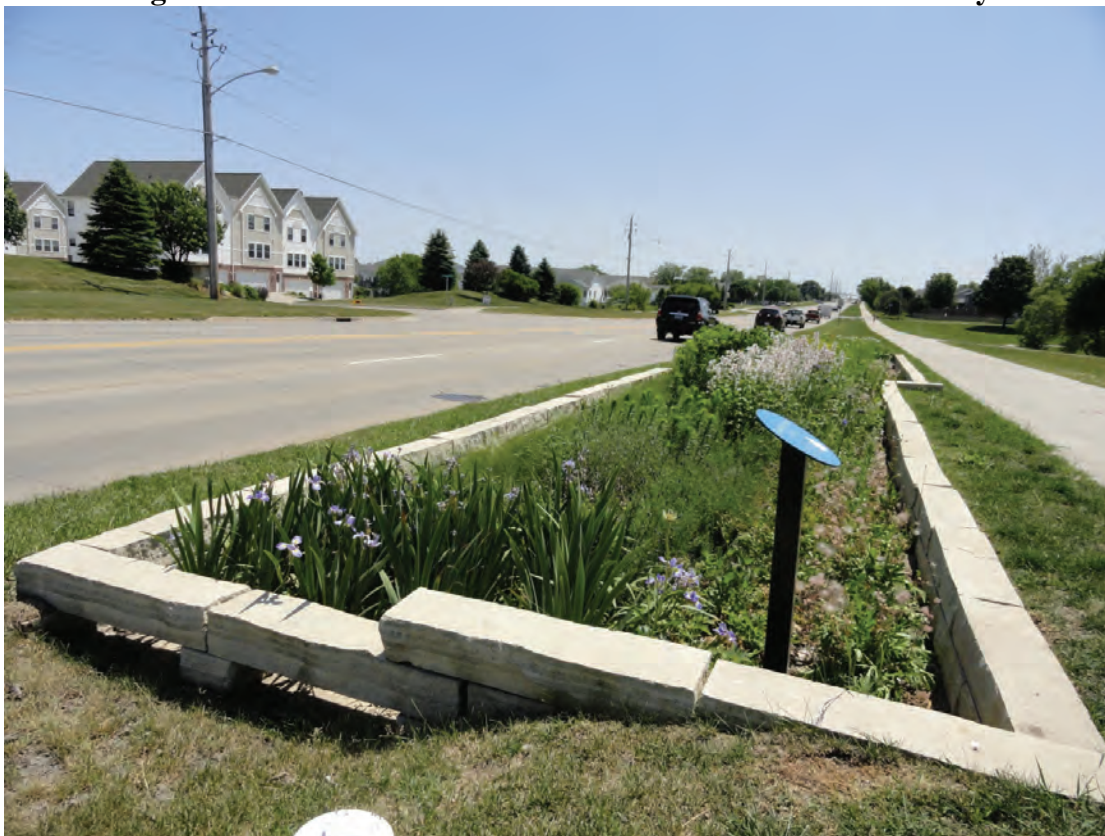
Figure 5.5: Bioretention units at Summerbrook Park in Ankeny
